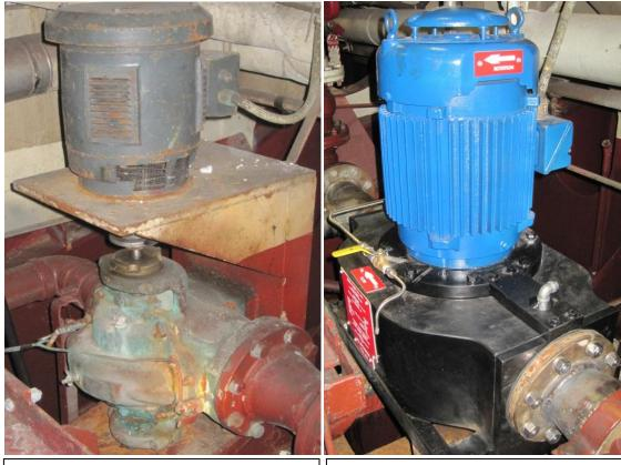
Figure 5. The old design Metallic Double-Suction Pump which is subject to corrosion Figure 6. The new design of a SIMSITE® Single-Suction Pump which Never Corrodes in Sea Water!
