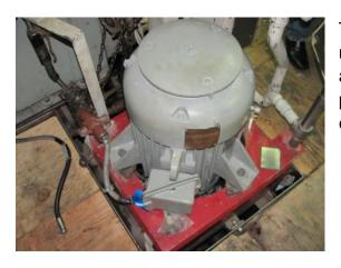
The **SIMS** MCM Seawater Fire Pump is mounted vertically onboard the Navy vessel and must fit into extremely tight space. The pump must not only corrode, but must also be completely non-magnetic and light weight.
