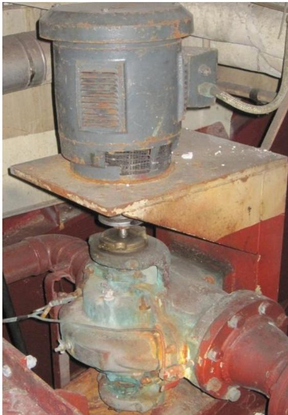
**Figure 5. The old design Metallic Double-Suction Pump which is subject to corrosion**
