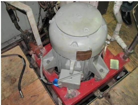
The **SIMS** MCM Seawater Fire Pump is mounted vertically onboard the Navy vessel and must fit into extremely tight space. The pump must not only corrode, but must also be completely non-magnetic and light weight.
