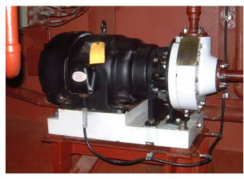
The above pumps are installed on NAVY Vessels for the Reverse Osmosis Systems (RO), which convert salt water to fresh water. These SIMSITE® Pumps will NEVER corrode in salt water!
